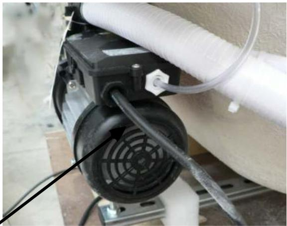
Check Capillary pipe is attached to on/off button and pump
